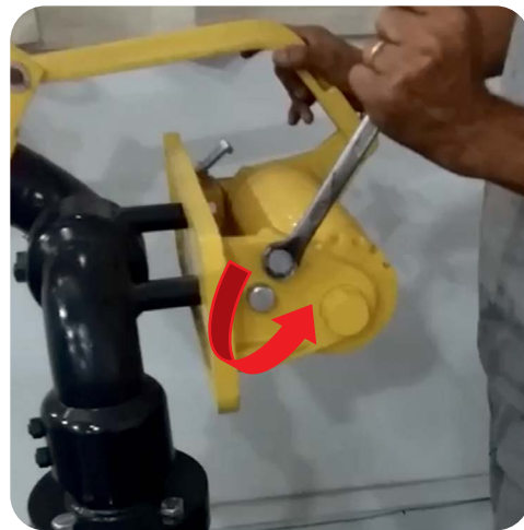
Image 7. Loosen the upper screw.
