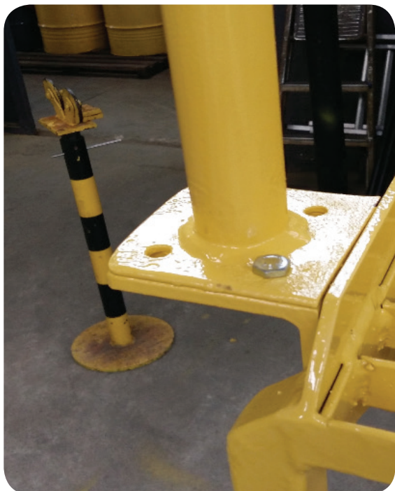
Image 4. Handrail footing secured to the base.
