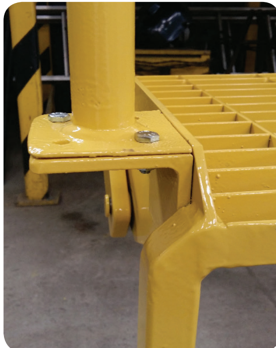
Image 5. Footing secured by four cap screws.
