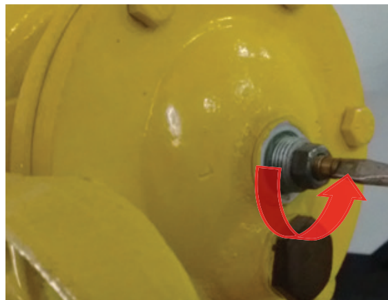
Image 17. Turn counter-clockwise for a faster shut-off.
